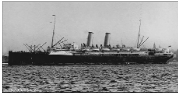
The Orient Line's SS Osterley ; 12,129 tons, 14,000HP, twin screws, 18 knots. Built 1909 by London & Glasgow Eng & Iron Shipbuilding Co.
